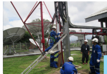
Fig. 1 Electricity Transmission Lighting Protection Installation Pekanbaru – Duri Riau (ITB-PLN).
