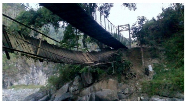
Fig. 2 The old bridge and the new one.
